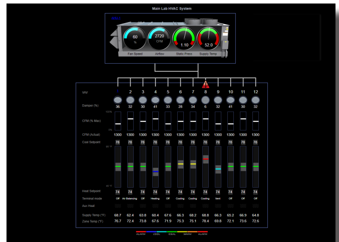
Lab HVAC System Screen
