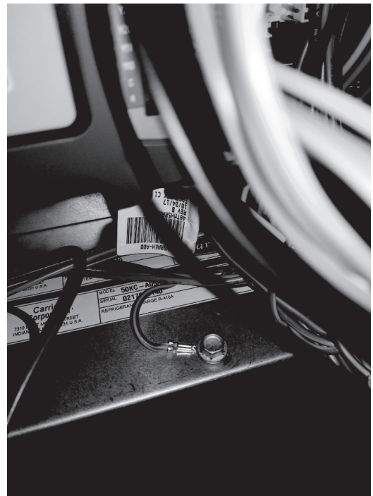
Fig. 12 — Connect Ground Wire From Controller
