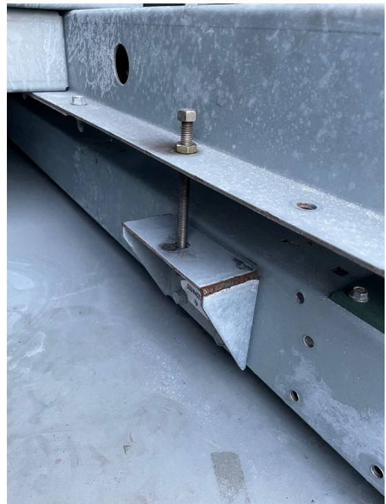
Fig. 52 — External Spring Compression Bolt
