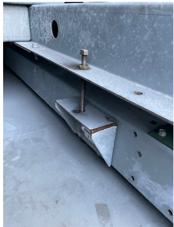
Fig. 51 — External Spring Compression Bolt
