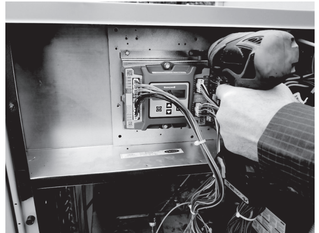
Fig. 10 — Mount Controller Assembly in Unit Control Box
