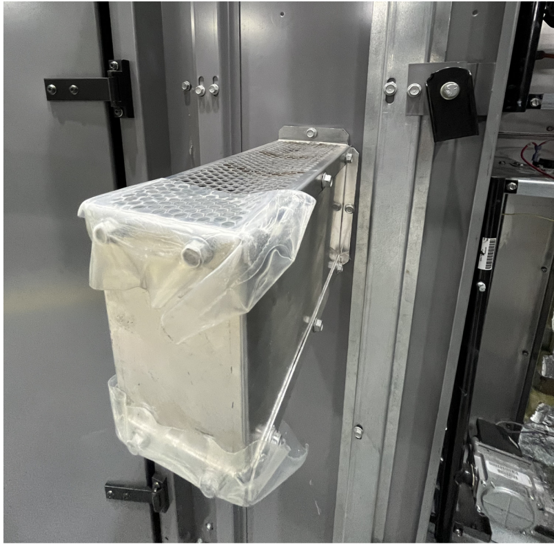
Fig. 3 — Flue Exhaust Hood
