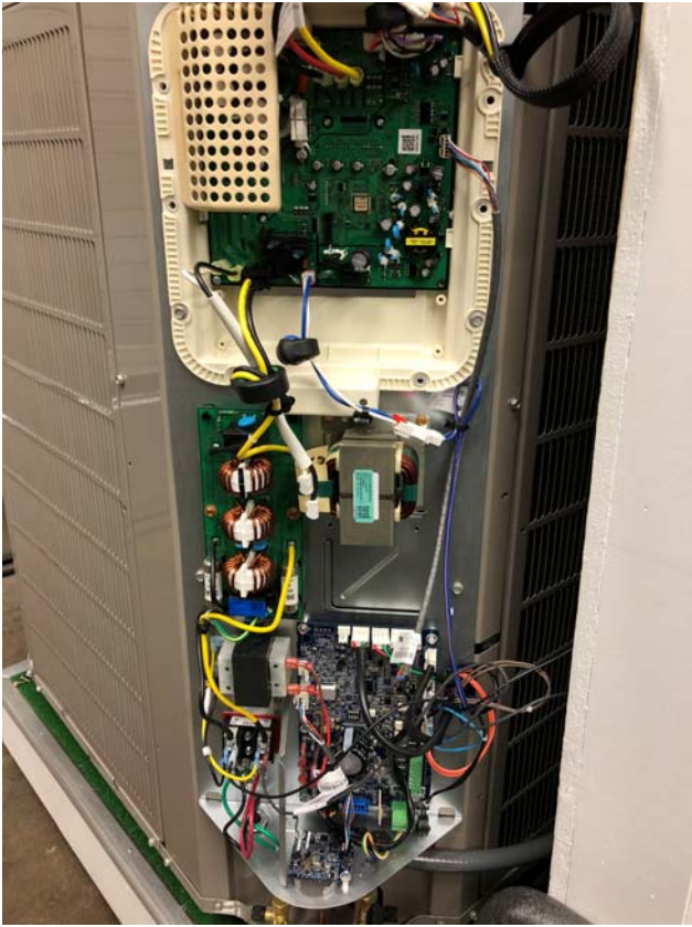
Fig. 19 – 2T/3T Control Box
