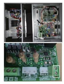
Fig. 10 — Connect the auxiliary heat wires
