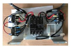
Fig. 13 — Circuit Breaker Label Placement
