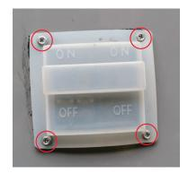
Fig. 15 — Fasten the resilient cap
