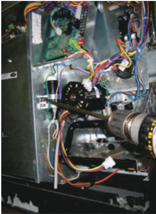
Fig. 29 – Removing Mounting Screw from Gas Manifold A210076
