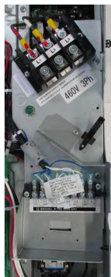
Close-up view of terminal block sub-assembly
