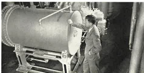
Onondaga Pottery, Syracuse, N. Y. Decalcomania. 1st Carrier Centrifugal Refrigeration Machine first placed in operation in 1922. Capacity, 67.5 tons.
