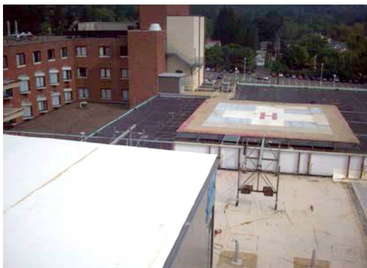
Figure 6 – Hospital Roof, Helicopter Landing Pad Close to O.A. Intakes
