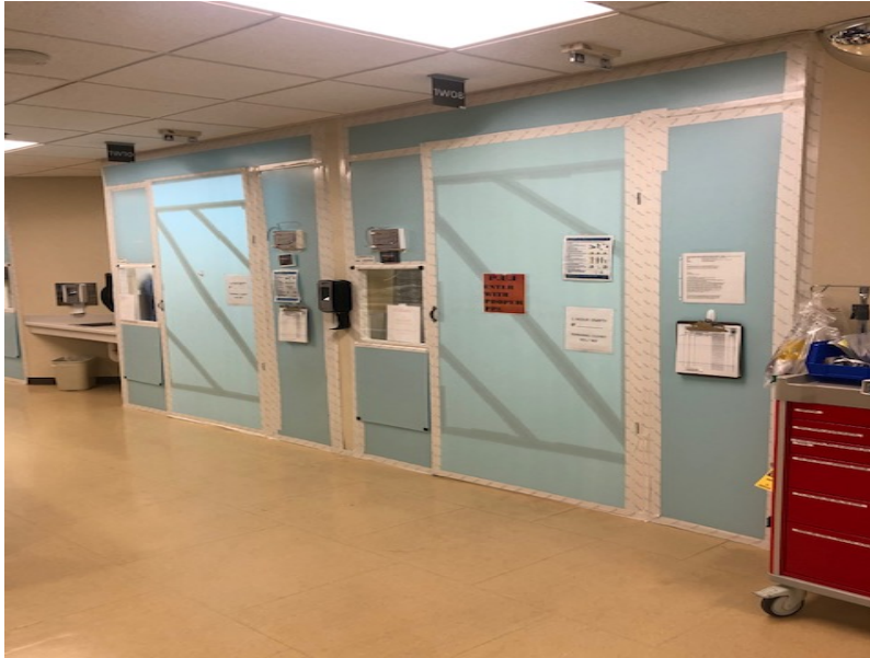
Photo 4: Temporary single negative patient rooms in ED. Photo Courtesy of Naval Hospital Camp Pendleton, Camp Pendleton, California
