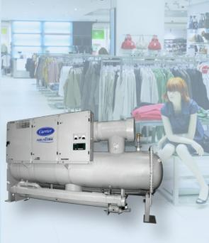
*Due to full load performance efficiencies up to 0.53 kW/Ton, and Integrated Part Load Values (IPLV) to 0.299, the Carrier AquaEdge® 23XRV water-cooled screw chiller provides economical comfort cooling for more than 500,000 ft<sup>2</sup> (46,451.5 m<sup>2</sup>) of retail space at tropical Mangabeira Shopping, located in João Pessoa, Brazil.*
