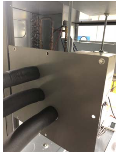
Fig. 56 - Knockouts and Line Sets
