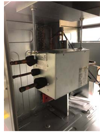
Fig. 54 - FS Unit Mounted to Threaded Rods
