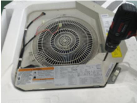
**Fig. 14 —Open Control Box Cover**
