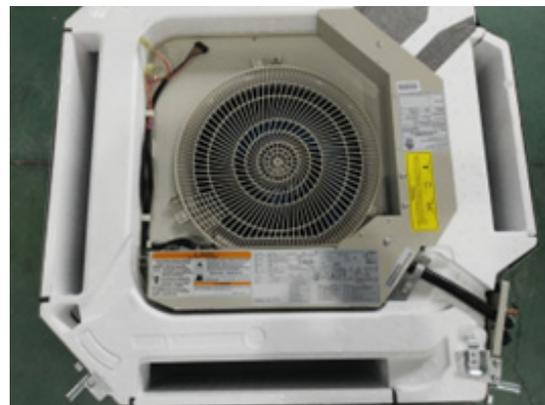
**Fig. 18 —Reinstall Control Box Cover**
