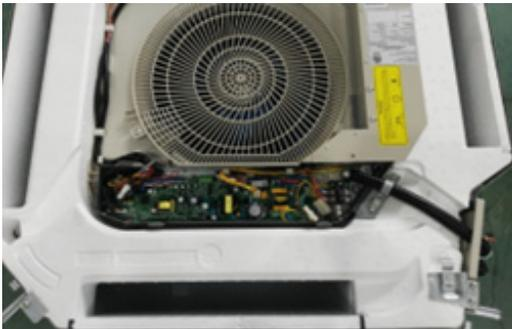
**Fig. 15 —Remove Clamp**
