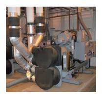
the heat they produce to a cooling tower for dissipation, the condenser water (up to  $138^{\circ}$ F) is pumped into the existing hot water loop, while also contributing chilled water to the cooling loop that serves a total of 767,121 ft<sup>2</sup> (71,267.9 m<sup>2</sup>) of space across multiple buildings.
