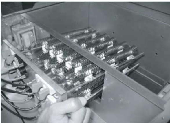
Fig. 3 —Slide Heater Kit into Slot and Secure with Screws
