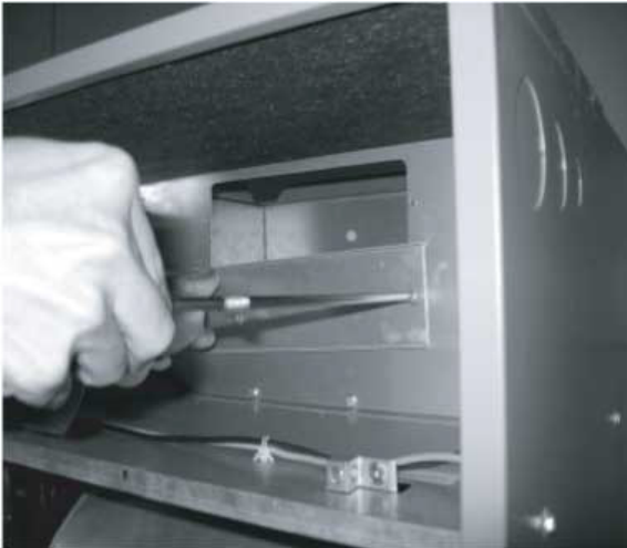
Fig. 2 —Remove Cover Plate from Air Handler
