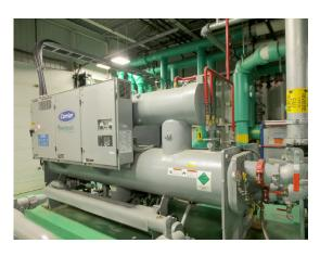
Evergreen® 23XRV water-cooled screw chiller, the first ever installed in Canada. The Evergreen 23XRV has met manufacturing parameters and delivered an energy savings of 80 percent over the previous unit. The chiller also uses the environmentally balanced refrigerant HFC-134a, which meets the environmental goals of the company.
