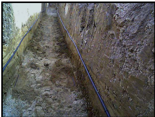
Fig. 5 Horizontal Closed Loop in Trench
