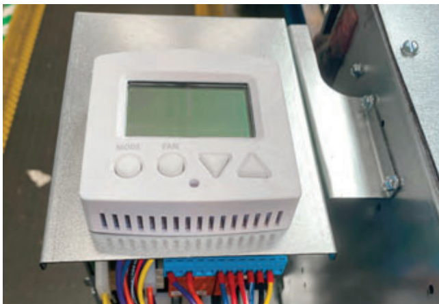
NOTE: Image depicts control box with thermostat mounted on 42VCA unit.
