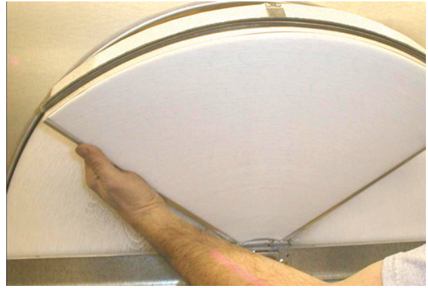
Fig. 34 — Segment Removal
