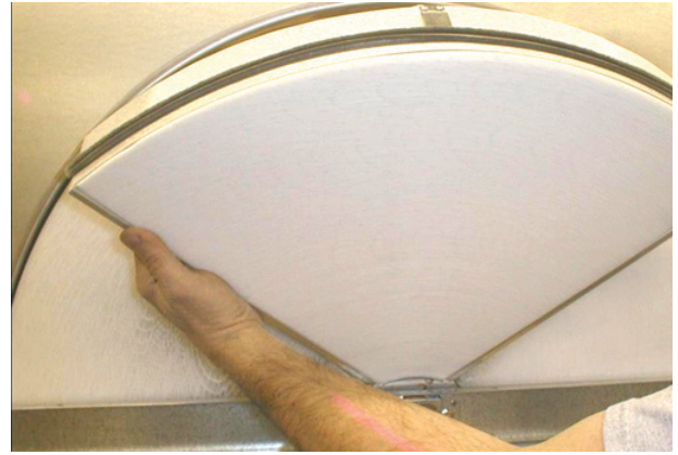
Fig. 31 — Segment Removal
