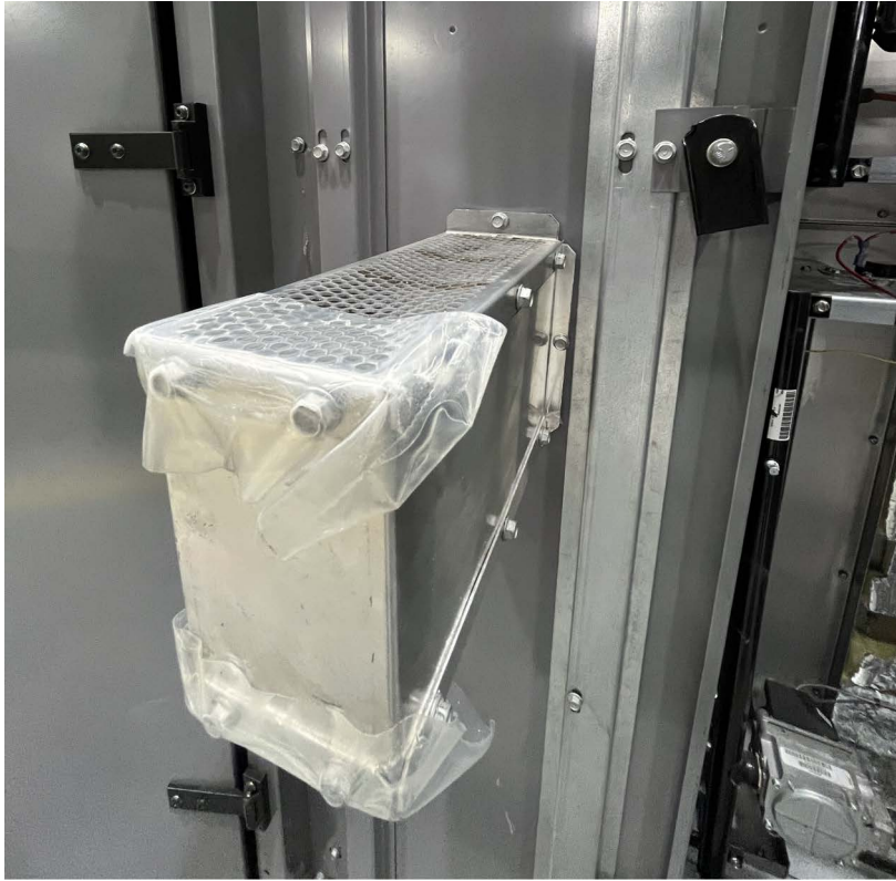
Fig. 4 — Flue Exhaust Hood
