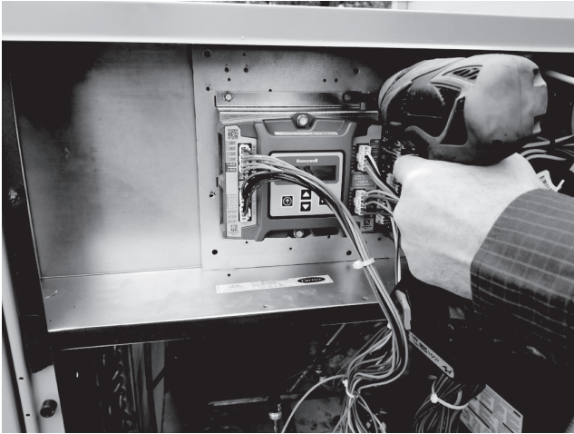
Fig. 9 — Mount Controller Assembly in Unit Control Box
