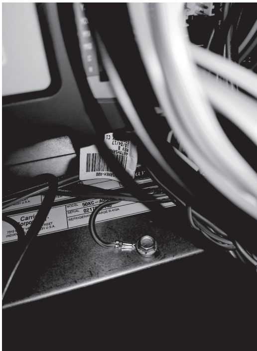
Fig. 20 — Connect Ground Wire From Controller
