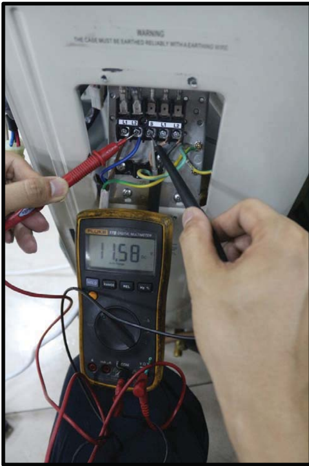
Fig. 23 – Test the DC voltage
