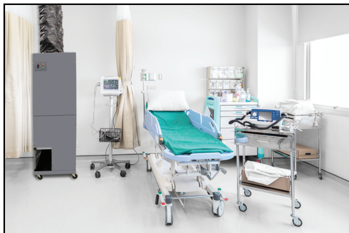
Fig. 2 – Room Setup Example for Negative Air
