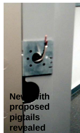
Proposed Door Hole Design- Electrical and Gas Left Side Entry
