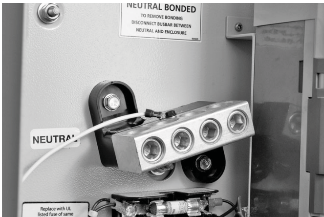
Figure 3.5 — RTSE Neutral Connection
