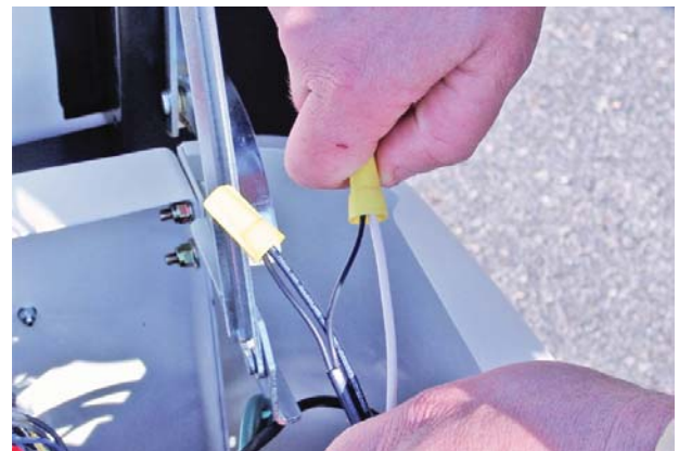
Figure 3.10 — Connection of Charger AC Input Wires in Generator Control Panel
