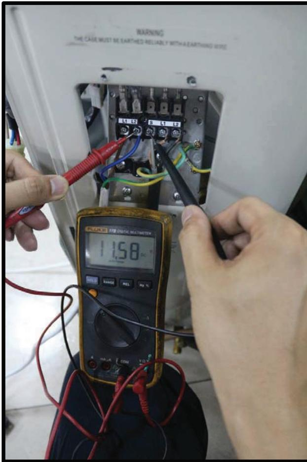
Fig. 27 – Test the DC voltage
