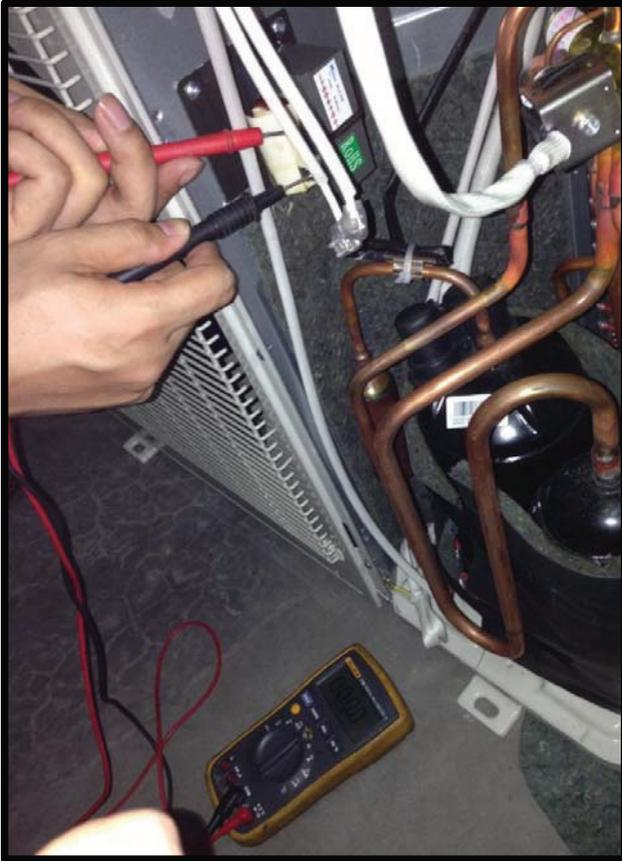
Fig. 28 – Test the resistance
