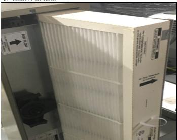
4. Remove the FEM (Filter Enhancement Module).
