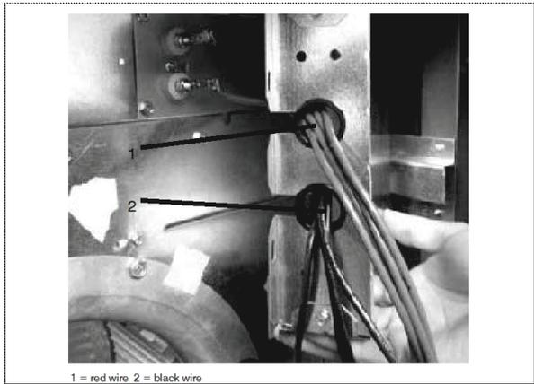
**Fig. 12 – Routing Red and Black Wires**
