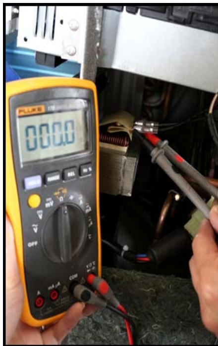
Fig. 31 – Test the Reactor Resistance
