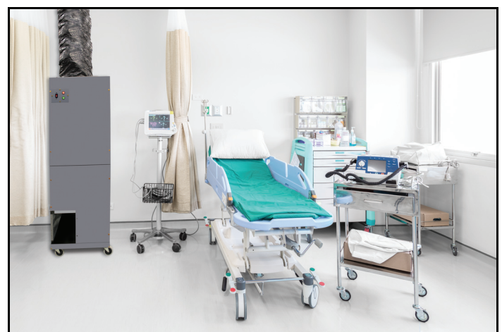
Fig. 2 – Room Setup Example for Negative Air
