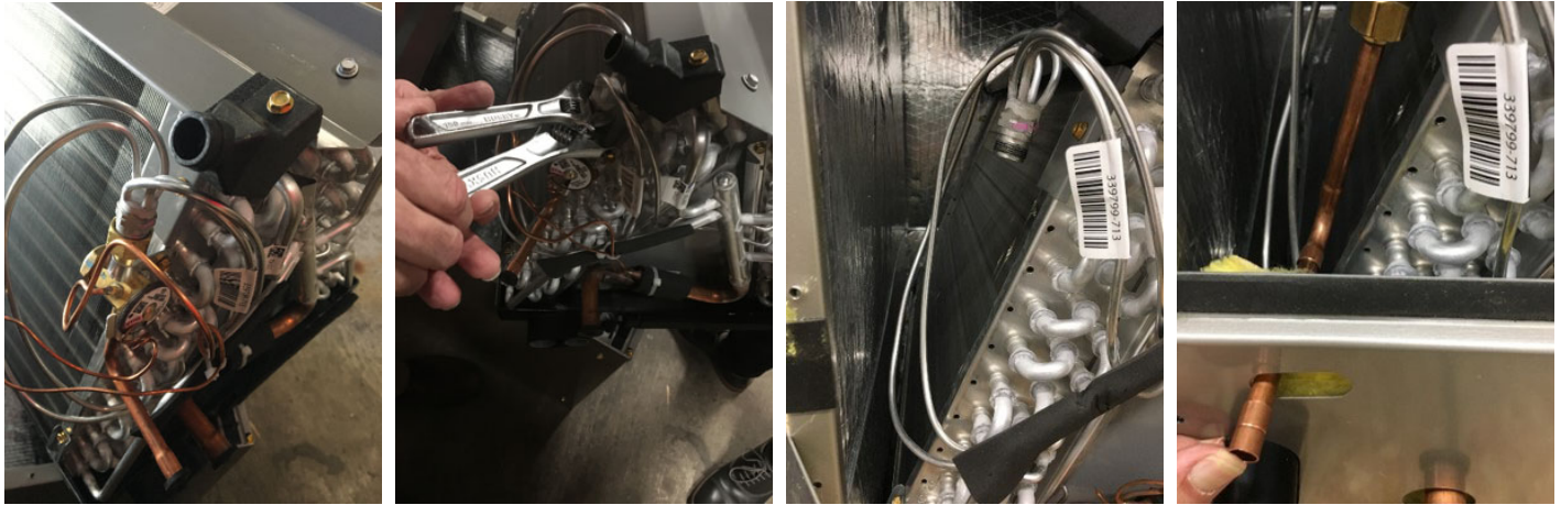
Fig. 14 — Piping Adapter Replacement
