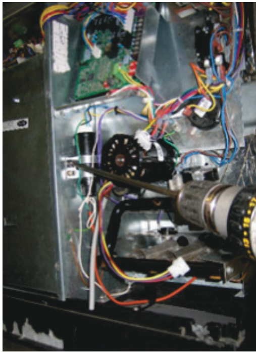
Fig. 32 – Removing Mounting Screw from Gas Manifold A210076
