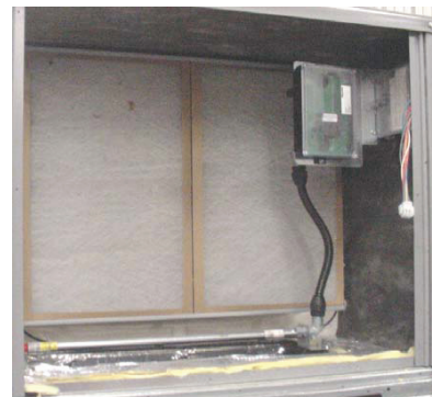
Fig. 24 - Return Air Sensor Operating Position
