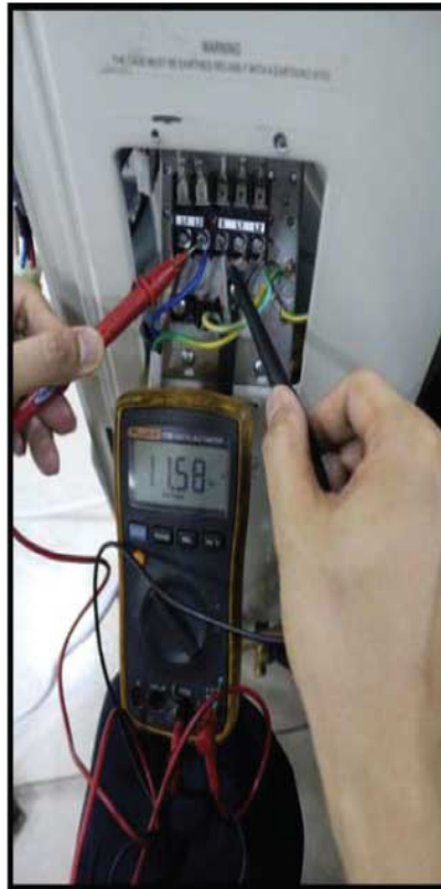
Fig. 40 —Test the DC Voltage
