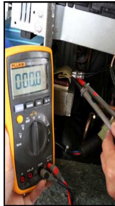
Fig. 17 —Test the Reactor Resistance
