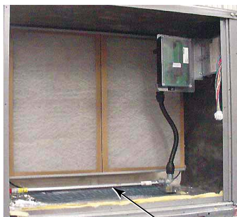
FIGURE 34 Return Air Sensor Operating Position
