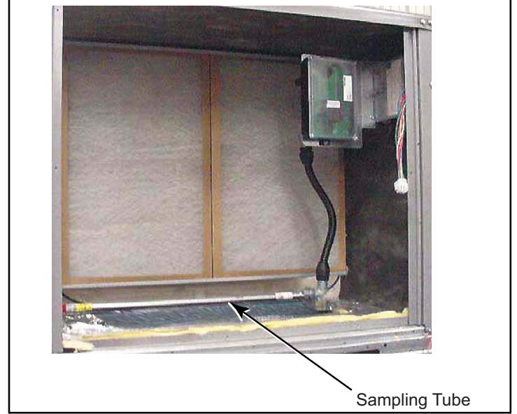
FIGURE 36 Return Air Sensor Operating Position
