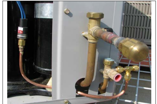
Fig. 1 — Low Ambient Pressure Switch
