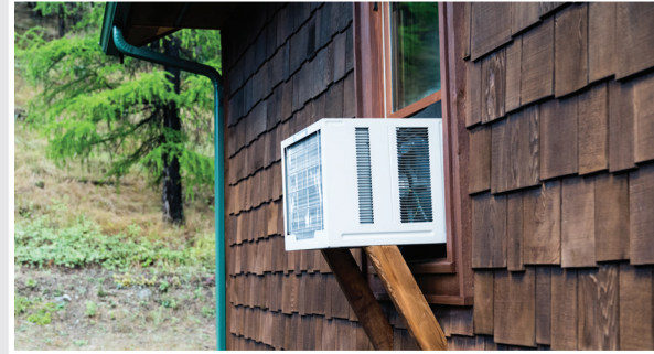
A2L refrigerants are safely used every day in millions of window units and car and truck AC systems.
