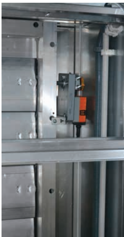
Damper motor inside and outside of the unit
