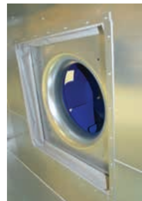
M0 fire class fan flexible connection
