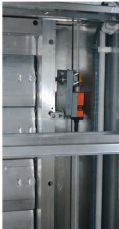
Internal or external damper actuator
