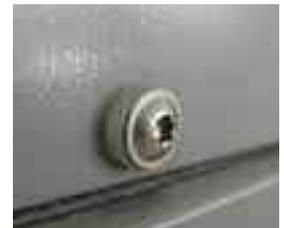
Stainless steel screw with plastic seal
