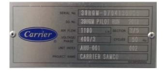
Sample of rating plate, above, contains the data for the AHU, such as Project Name, Section number, power
