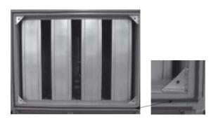
Use the pre-mounted corners for the final positioning of the sections and secure the corners with a bolt. The sections must be fully aligned.
