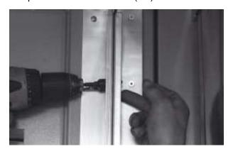
If there are more than two sections, repeat the procedure above. For an outdoor installation all external joints should be sealed.
