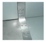
Remove the first two corners and mount the GI connection strip to the base. Remove the next two corners and mount the connection strip against the side wall. Repeat this for the other AHU corners.
