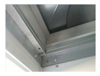
Ensure that the sealing tape supplied is fixed to one of the two sections, before moving the sections against each other
