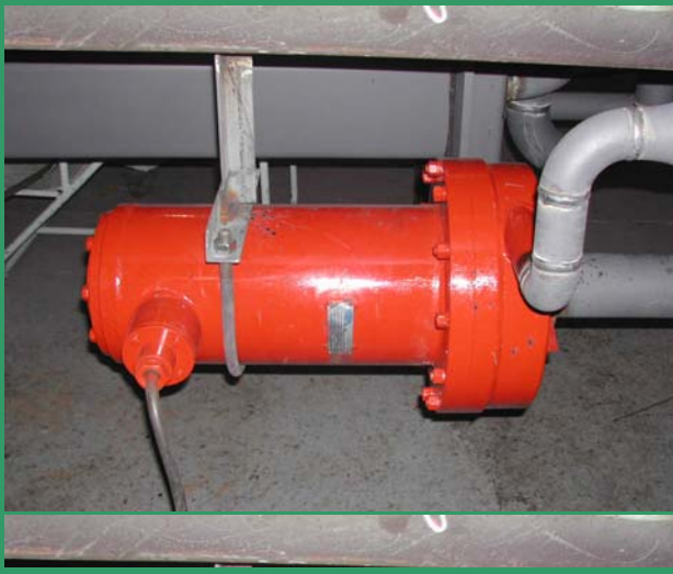
VIEW OF TYPICAL HERMETIC PUMP/MOTOR ASSEMBLIES
