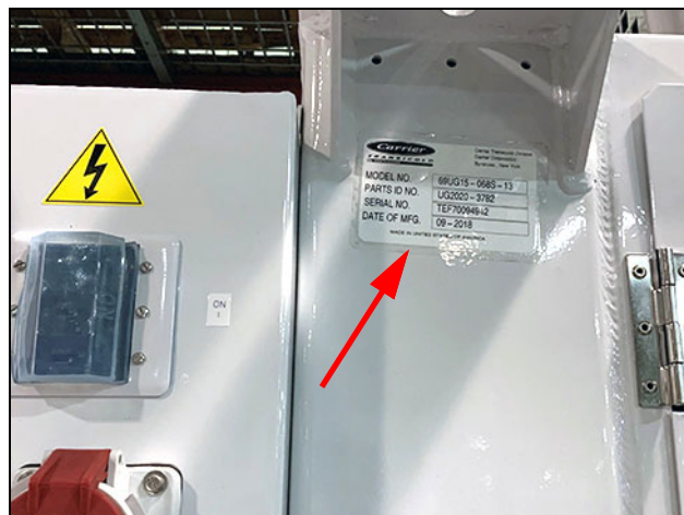
Figure 2.1 Label with Generator Set Identification
