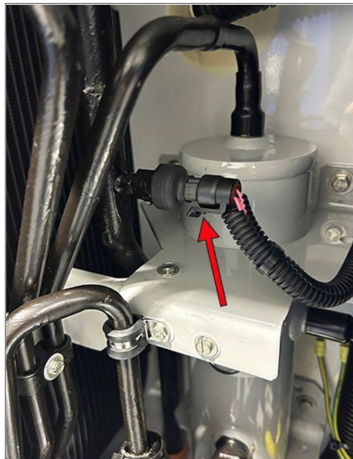
Figur 3.24 Afgangstryktransducer (DPT)
