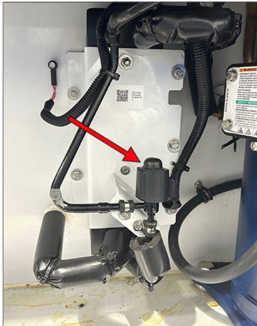
Figur 3.21 Economizer-ekspansionsventil (ECV)
